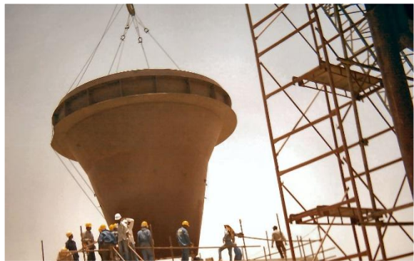
Bottom Cone (Conditioning Tower) – Installation
