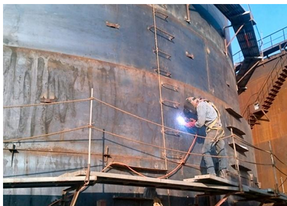
On-Site Tank Fabrication
