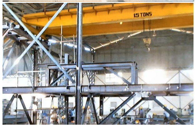
Steel Structure - Trial Assembly
