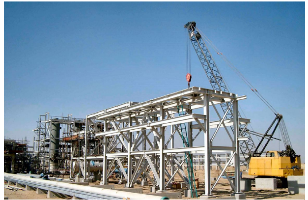
Steel Structure for Gas Gathering Plant
