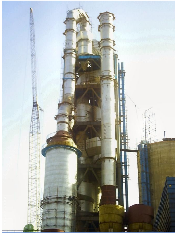
Pre-Heater Tower – Fabrication and Installation
