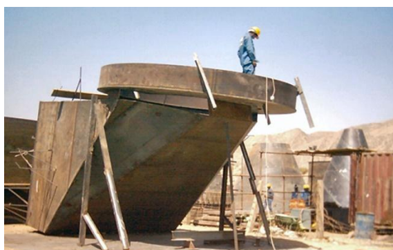
On-Site Fabrication Yard
