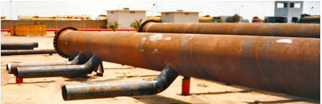
Fabrication of Piping Spool
