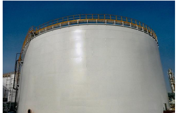
Biogas Digester Tank
