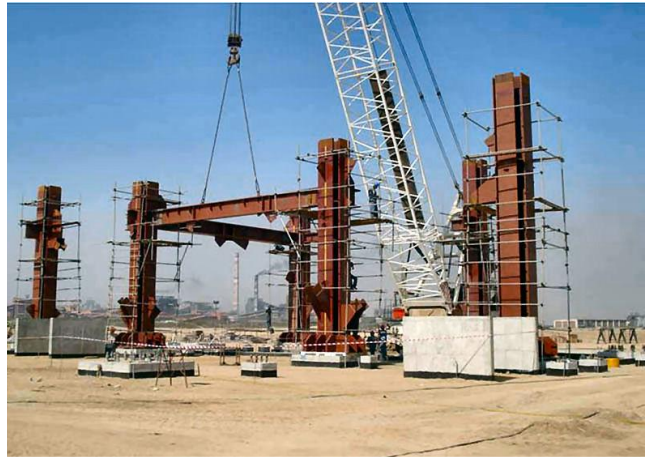
Erection of Steel Structure for DRI Furnace
