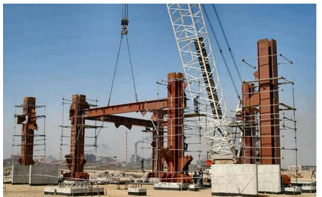
Steel Structure - DRI Furnace (Steel Mills)
