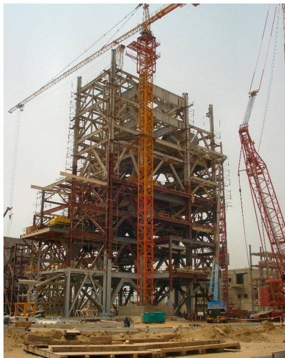
On-Site Steel Structure Fabrication & Erection
