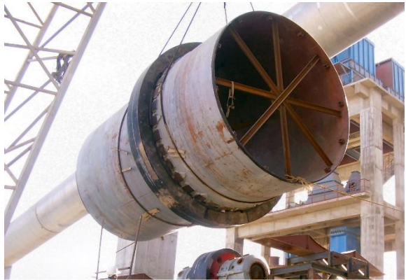
Kiln Shell – Installation
