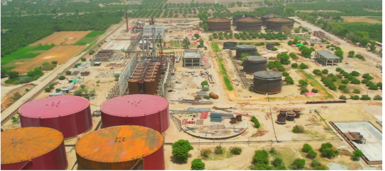
Complete Mechanical works of Ethanol Plant
