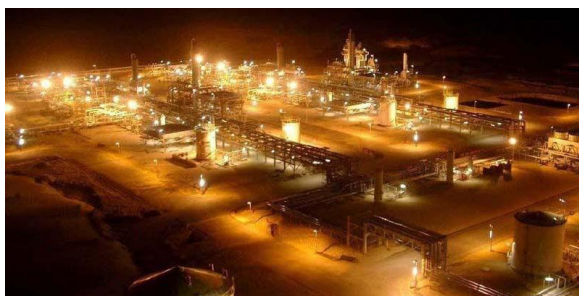
Steel Structure – Complete Plant
