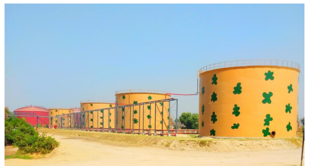
Alcohol Storage tanks
