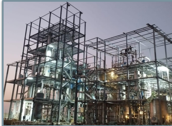
Multi Story Steel Structure for 200 TPD Fatty Acid Methyl Ester Plant
