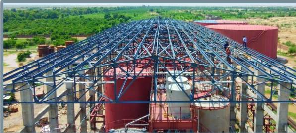
Steel Structure for Ethanol Plant
