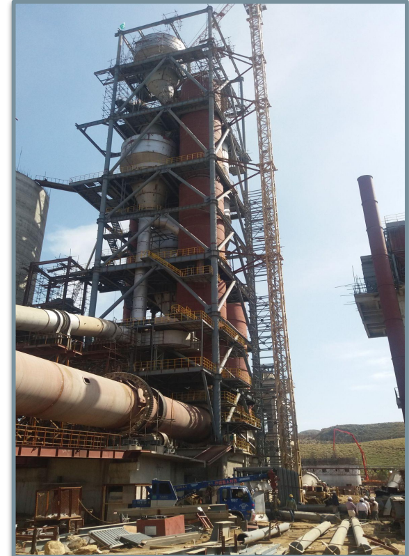
Steel Structure for Preheater Tower and Kiln
