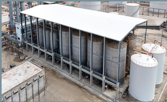
Prefabricated Shed for Fermentation House
