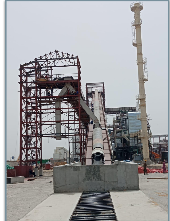
Steel Structure for Boiler Fuel Handling
