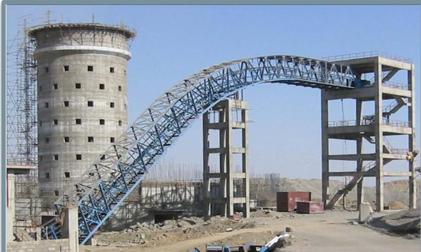
Truss for Clinker Handling System
