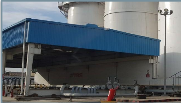
PEB for Oil Terminal
