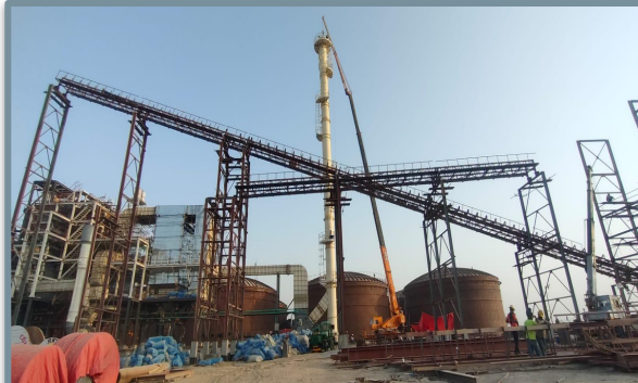
Steel Structure for Boiler Fuel Handling
