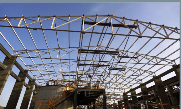
Steel Structure of Fermentation House for Ethanol Plant
