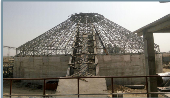
Clinker Storage Shed
